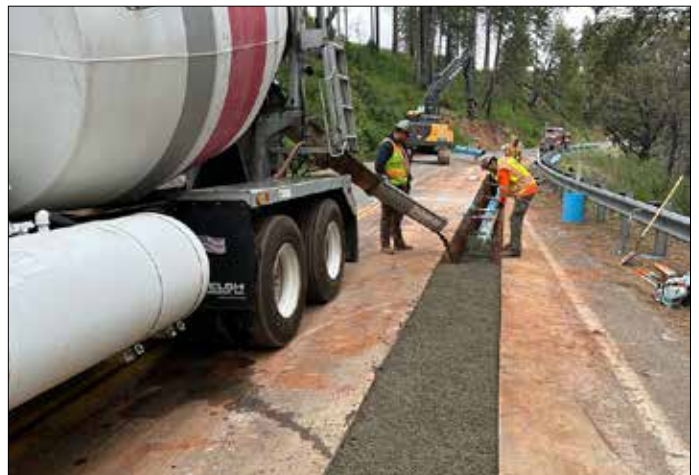
Above: Concrete pads for PID’s two new steel water tanks; each will hold 1.5 million gallons of water. Below: Work continues on the Zone A pipeline installation to create a redundant water supply for customers in case of problems with the existing line.
