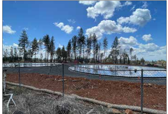
Above: Concrete pads for PID’s two new steel water tanks; each will hold 1.5 million gallons of water. Below: Work continues on the Zone A pipeline installation to create a redundant water supply for customers in case of problems with the existing line.
