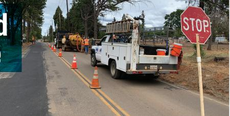
PID's crews are busy replacing service lateral lines (those from the PID main lines to homes) throughout the district. Here a crew works on Foster Road.
