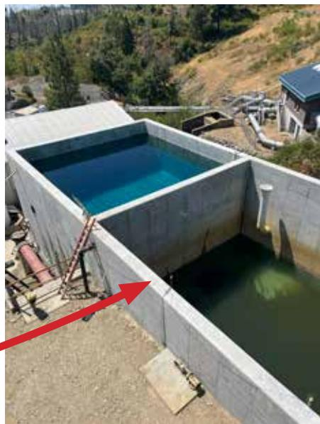
*Left: PID's new equalization tank allows “wash water” from Treatment Plant filters to be held before being pumped to the district's settling ponds. This is not treated water for our customers' use, but water that is being prepared for the settling ponds.*
