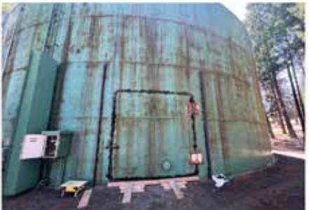
*Top left: Workers first cut into tank to create a door large enough to drive a forklift through.*
