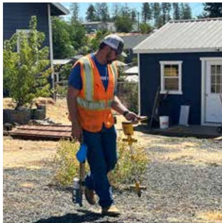
**PID's Aaron Ropp uses a locator to spot and mark underground PID water lines so a contractor doesn't accidentally dig into the line.**
