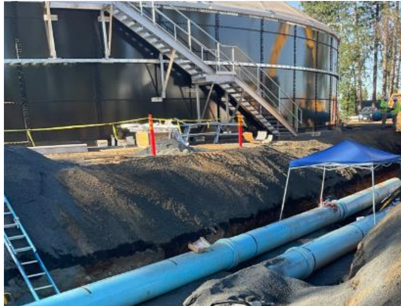
Figure 1: Tank B-2 Sidewall and Stairway with the 24" fill and draw lines in the foreground
